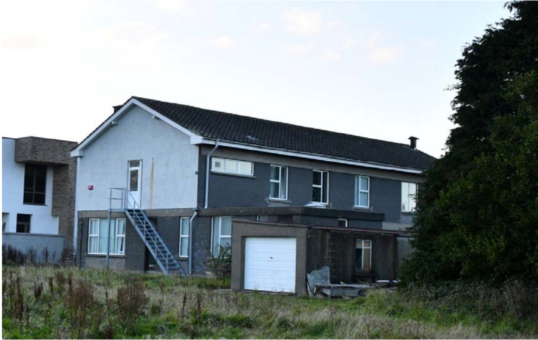
Plate 1. Existing building on site.
